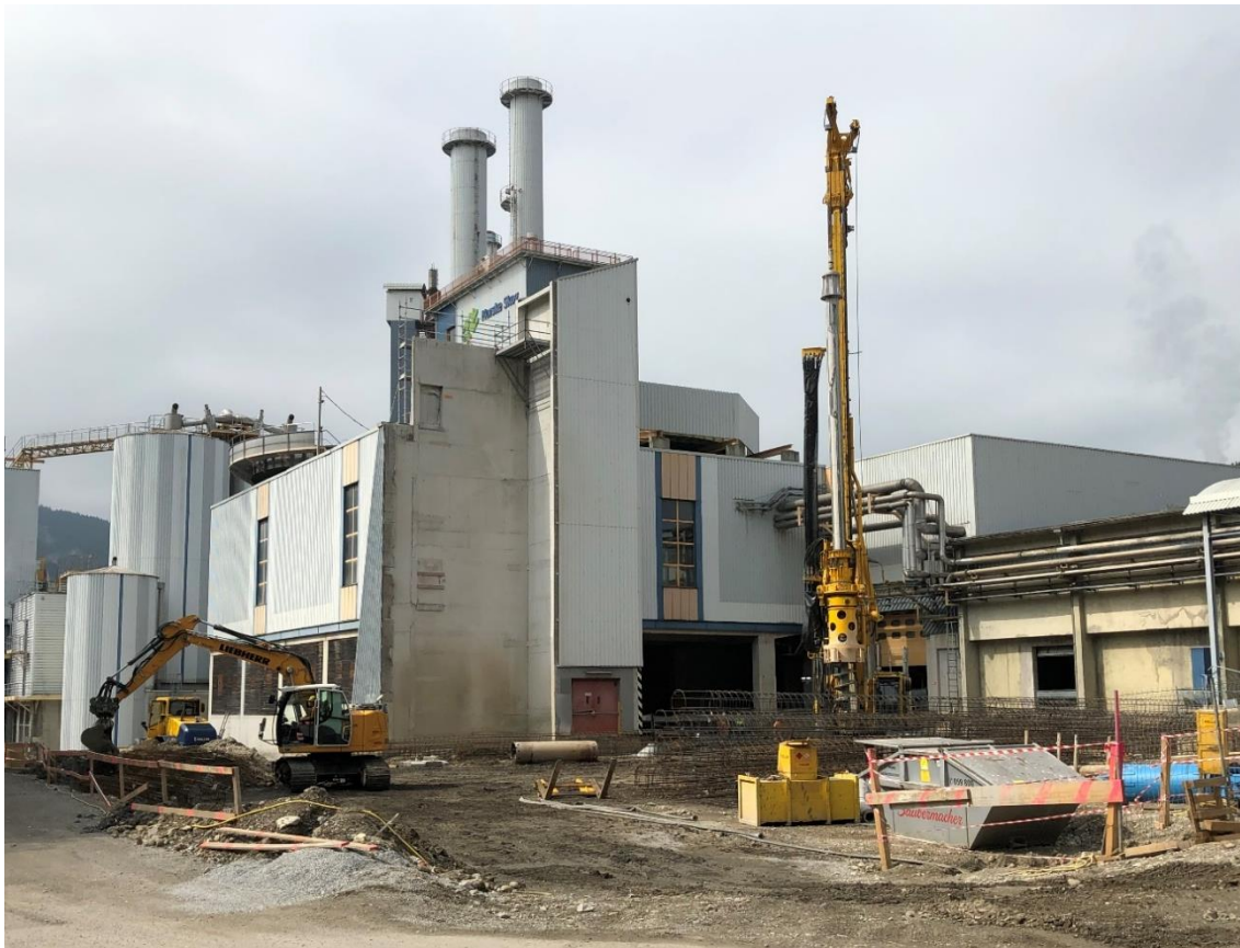
Waste to energy plant being installed in Bruck, Austria
