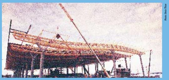
The terminal building at Oslo's new main airport, Gardermoen, is being built of Norwegian natural materials - wood and stone. The huge laminated wood beams were produced by Moelven Industrier; the automatically strength-graded sawn timber of which they are made was supplied by Norske Skog sawmills, Soknabruket and Våler Skurlag.
